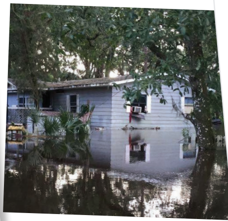
This Florida house was one of many ravaged by flooding.
